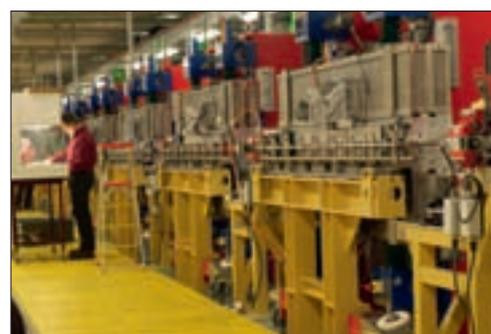
**Figure D.** FEL I undulators installed in the undulator hall.
